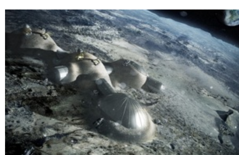
Concept sketch of multi-dome, inflatable Moon base covered in 3D printed lunar regolith.
