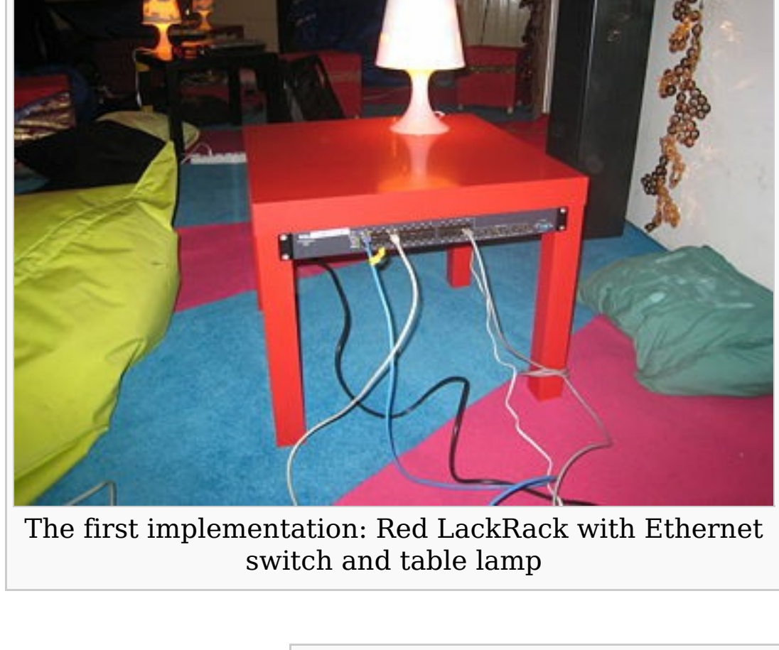
The first implementation: Red LackRack with Ethernet switch and table lamp
