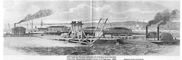
The 'Floating Railway', opened in 1850 as the first roll-on roll-off train ferry in the world.
