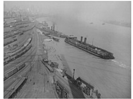
Classification yard and two docking train ferries in Detroit, April 1943. A third ferry slip can be seen at the bottom of the photograph.
