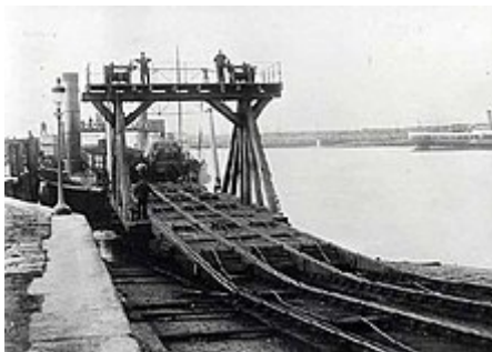
Bouch's ferry design. Note the adjustable ramp.
