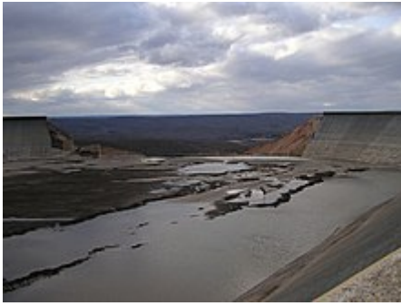
In 2005, a large section of the upper reservoir failed, draining over 1 billion US gallons (3.8 gegalitres) of water in less than half an hour.
