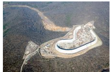
Aerial photo shows reconstruction progress in late November 2009
