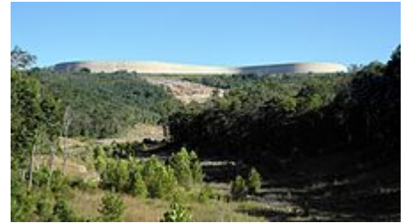
The completed replacement reservoir, viewed from the scour created by the collapse of the original.
