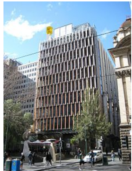
Council House 2 . Wind towers in concrete canyon to the left.
