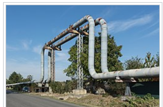
Expansion loop on heating pipeline
