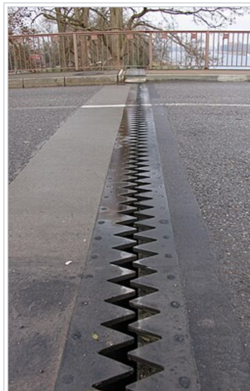
Expansion joint in a road bridge used to avoid damage from thermal expansion.
