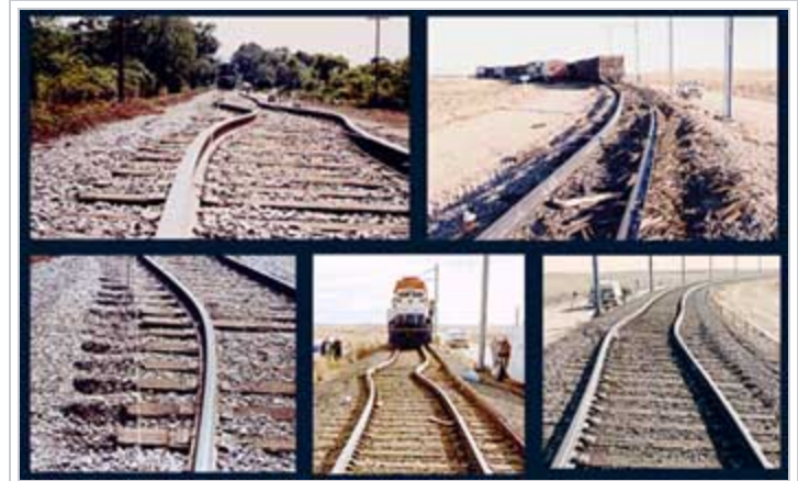
Thermal expansion of long continuous sections of rail tracks is the driving force for rail buckling . This phenomenon resulted in 190 train derailments during 1998–2002 in the US alone. [47]
