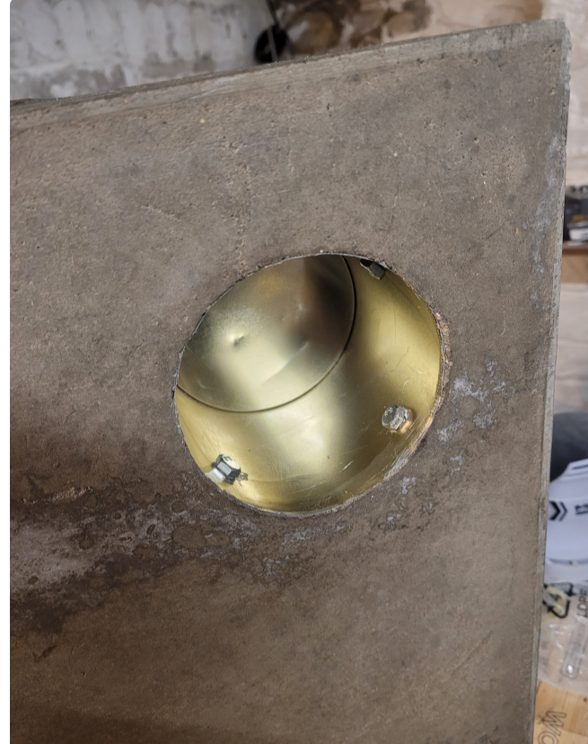
Integral plant pot is a tin set into the concrete
